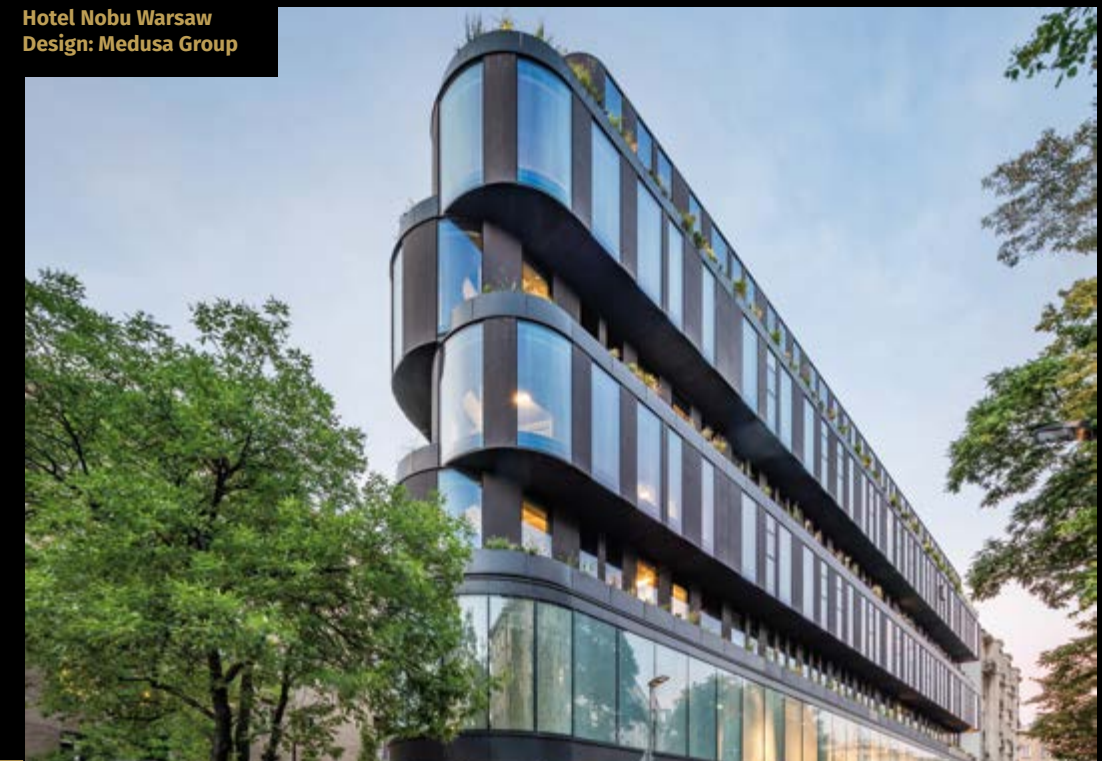
Aluprof systems: MB-SR50N EFEKT mullion and transom façade system, MB-SR50N EI EFEKT mullion and transom façade system, MB-SR50N OW tilt-and-slide window system, MB-86 SI and MB-86 ST thermally broken window and door system, MB-SKYLINE sliding door system with concealed frame, MB-78 EI fire-rated partition system with doors
