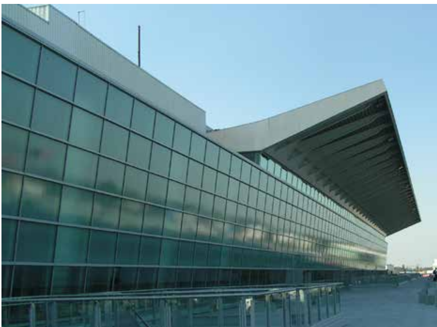
Warsaw Chopin Airport, Warsaw design / arch. Pierluca Roccheggiani, arch. Paweł Czaplicki
