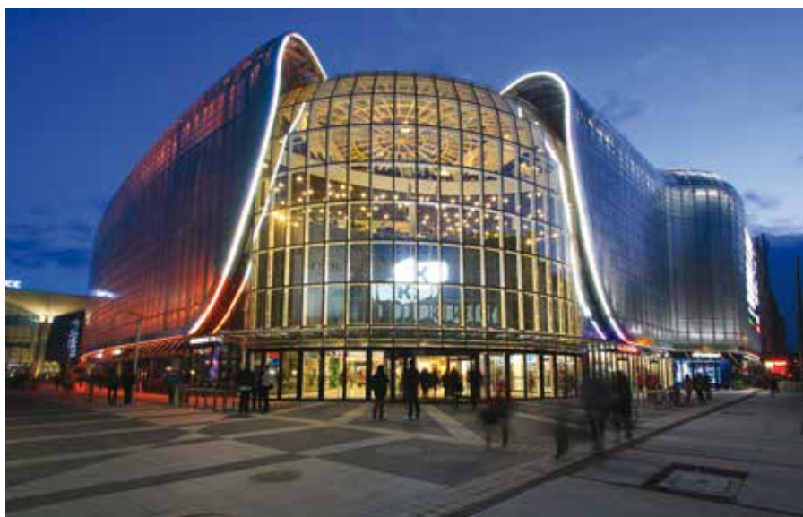
Katowice Gallery, Poland design / SUD ARCHITECTES
