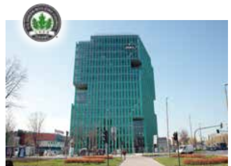
Alma Tower, Cracow - LEED PLATINUM
